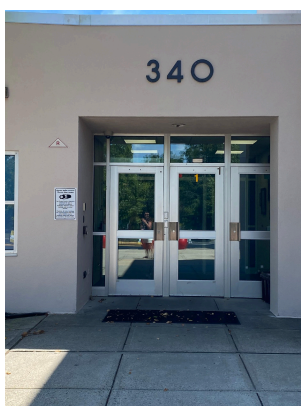
Kindergarten — Main Entrance
